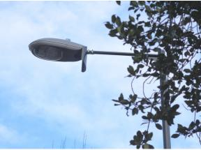
Below: Typical efficient full-cut off street lighting, with shields
