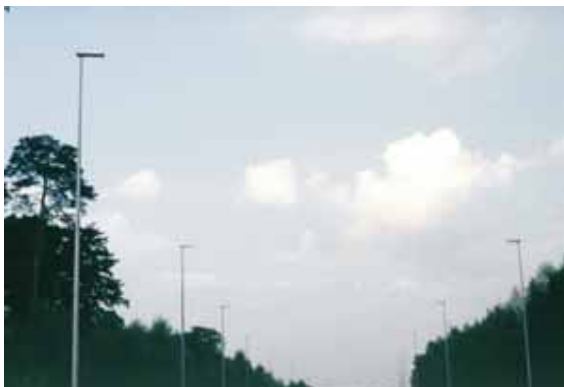
Full cut-off lights on the M27 motorway C. Baddley
